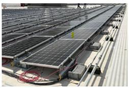
JMT provided design support services along with mechanical and electrical engineering for this new, free-standing photovoltaic canopy system with EVCS charging and a battery storage system.
